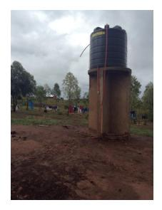
Nyakasimbi Secondary School was fortunate enough to acquire a borehole in early 2019. It was in the unusual position of having access to water, but no way to pipe it out of the ground. Action in Africa has contributed to the cost of water pipes and a tank on a tower for gravitational distribution (pictured above).
