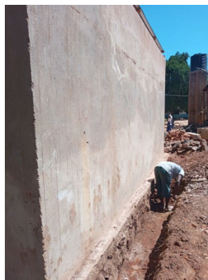
External plastering of the tank
