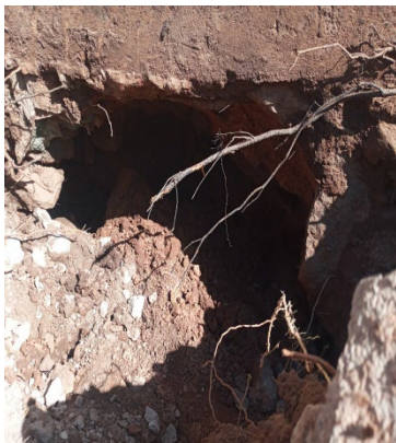
Scour under the main tank
