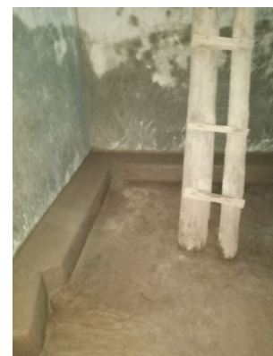
Internal plastering
